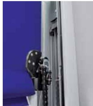
*After the manual operation of the control, the door moves downwards into the closed position. All of the systems regenerate completely automatically: door curtain and closing edge are guided back to the frame by means of the tensioning ropes, the snap-in connections are connected again when the end position is reached.*
